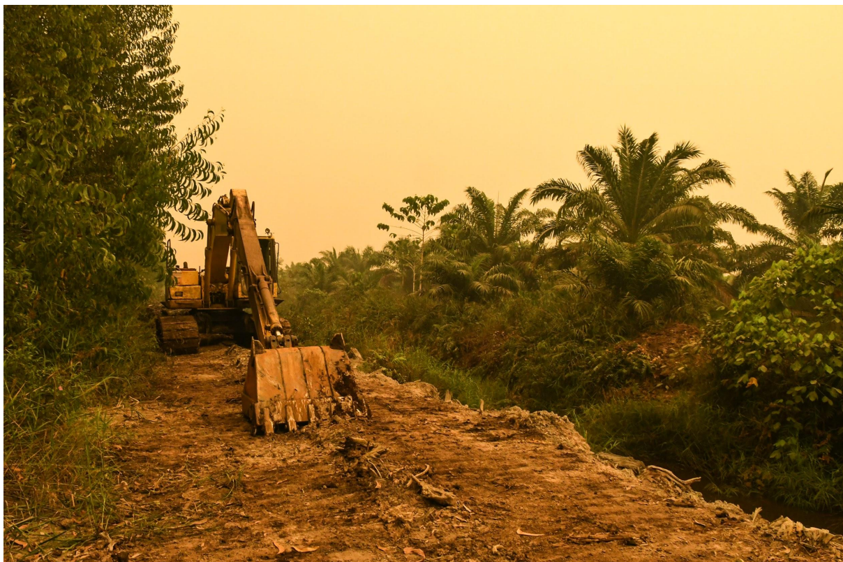
21 September 2019, PT Kaswari Unggul, 1°17'50.699" S 103°45'41.92" E: An excavator at work in the haze from peatland fires in the PT Bukit Barisan Indah Prima concession in Jambi. The plantation company is currently facing civil court action. PT Kaswari Unggul is named as a supplier to Unilever, Mondelēz, Nestlé and Procter & Gamble as well as Wilmar, GAR and Cargill.
