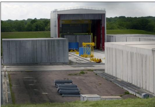
However, only after 10 years of operation, tritium leakage from CSA has been identified in the underground aquifer, while the site has no license to discharge any radioactivity. Furthermore, in a recent incident, a concrete cell containing the waste cracked under excessive pressure. This was assessed as a generic design failure by the French nuclear authority ASN in a letter of May 24<sup>th</sup> 2006 (see letter in annex). By the end of 2002 it is estimated there was as much
