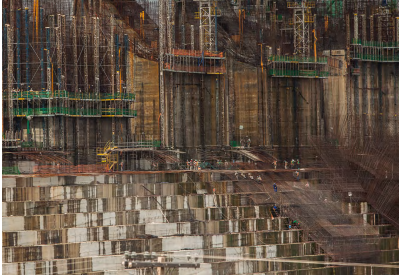
Construction of the Belo Monte hydropower complex, Pará State.. © Carol Quintanilha/Greenpeace
