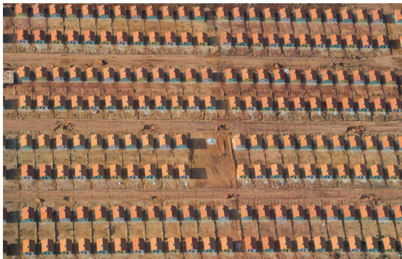
Housing for construction workers near the Belo Monte hydropower complex, Pará State © Daniel Beltrá/Greenpeace
