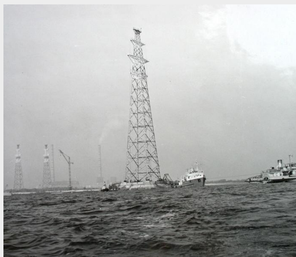
Power line supports were built on the shore, after which they were towed to the installation sites in the Kakhovka Reservoir. Image source: Provided from a private archive.
