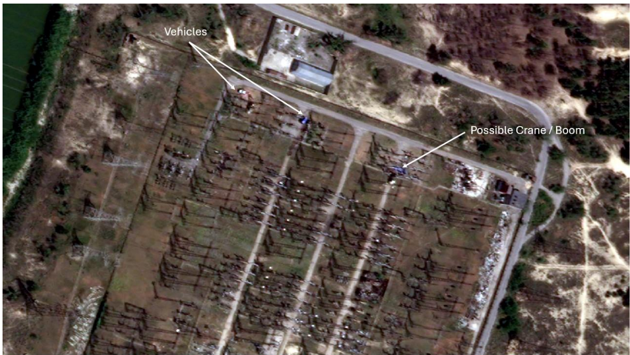
Fig.5 – Activity in Ferosplavna 330kV open switchyard area on 6 June 2026.
