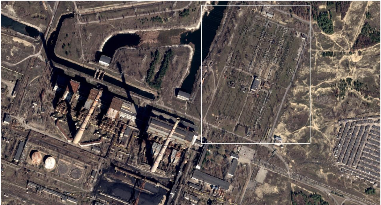
Fig. 1 - Location of Ferosplavna 330kV open switchyard. Image dated 15 October 2025
