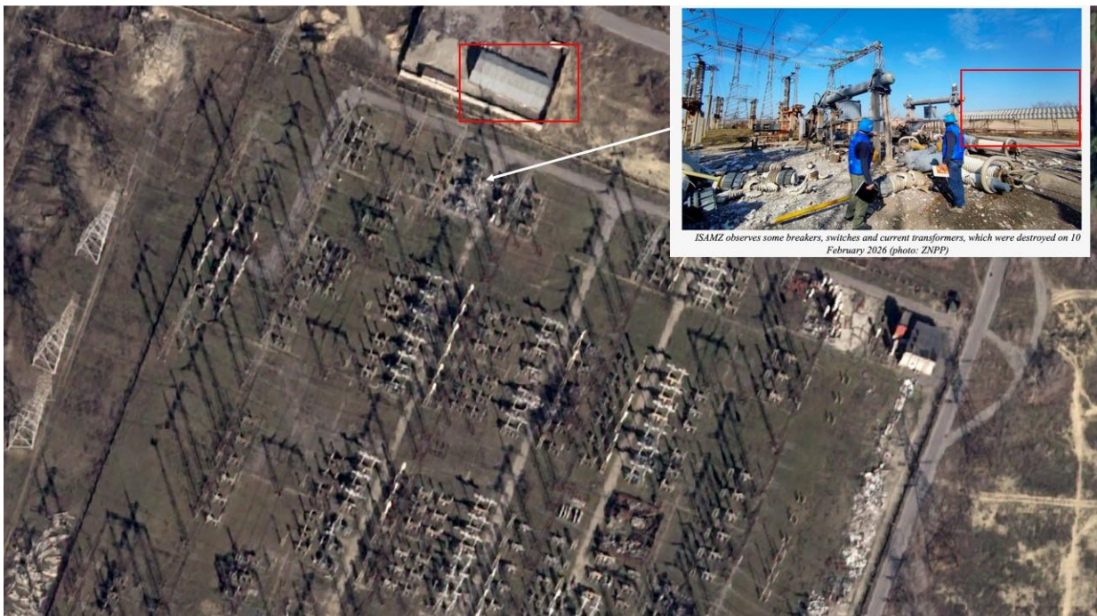
Fig. 3 – Area with debris dated 27 February 2026.
