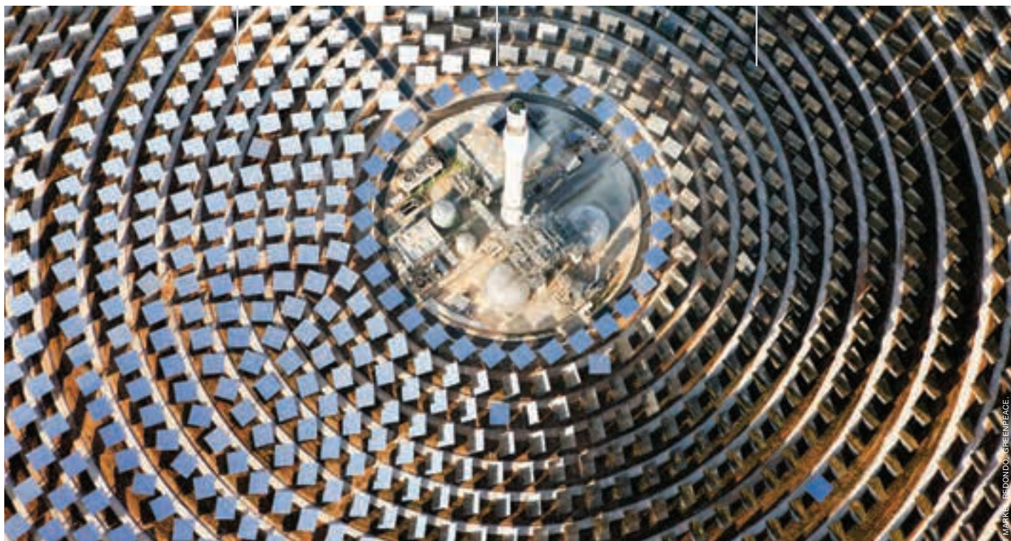
IMAGE GEMASOLAR, A 15 MW SOLAR POWER TOWER PLANT, SPAIN.
