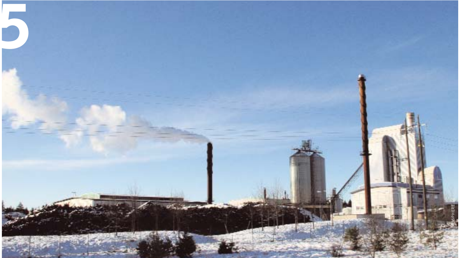
image BIOMASS ENERGY PLANT NEAR VARNAMO, SWEDEN.
