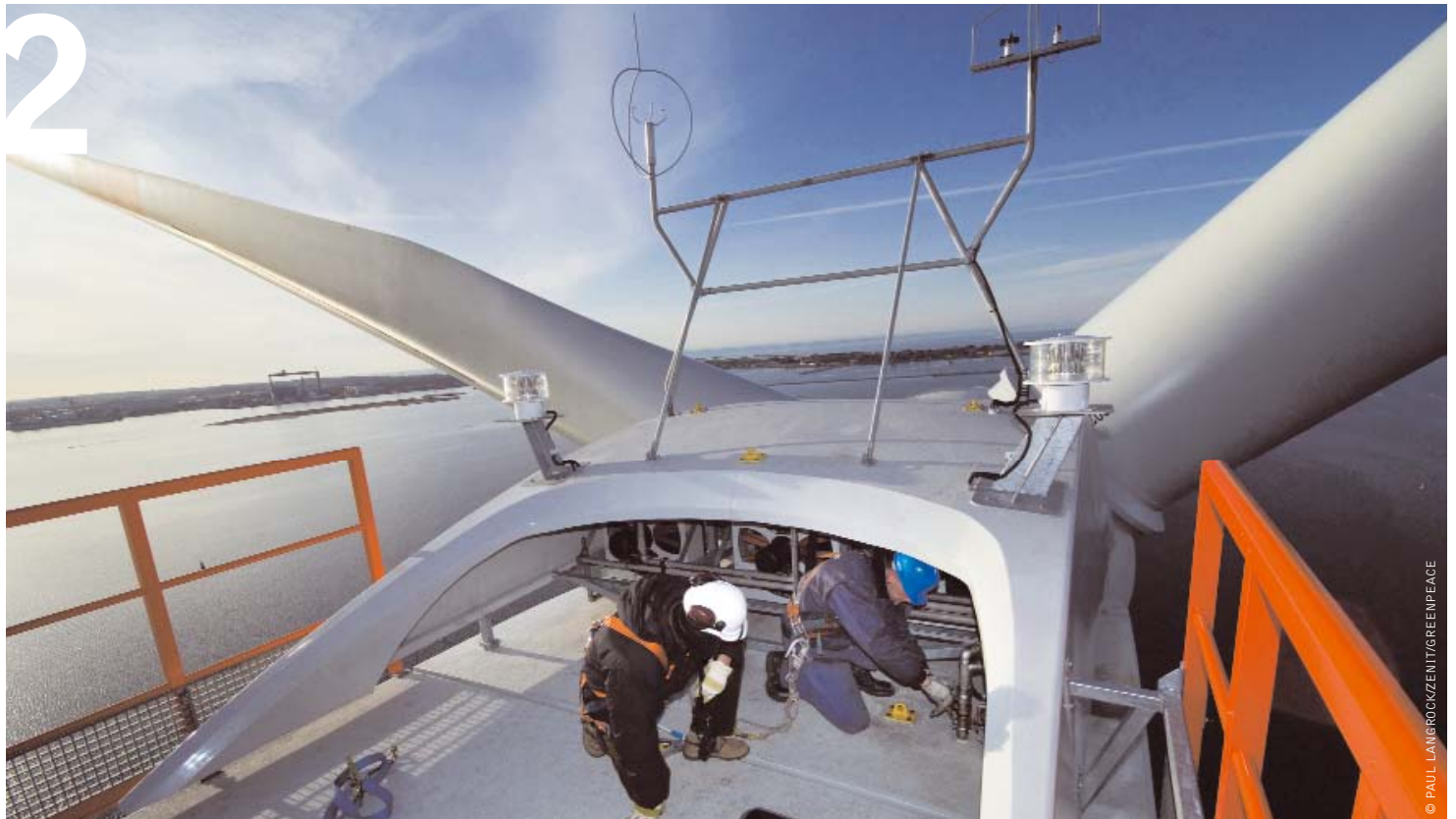
image TWO TECHNICIANS WORKING INSIDE THE TURBINE OF TEST WINDMILL N90 2500, BUILT BY THE GERMAN COMPANY NORDEX, IN THE HARBOUR OF ROSTOCK. THIS WINDMILL PRODUCES 2,5 MEGA WATT AND IS TESTED UNDER OFFSHORE CONDITIONS. AT LEAST 10 FACILITIES OF THIS TYPE WILL BE ERECTED 20 KM OFF THE ISLAND DARSS IN THE BALTIC SEA BY 2007. TWO TECHNICIANS WORKING INSIDE THE TURBINE.
