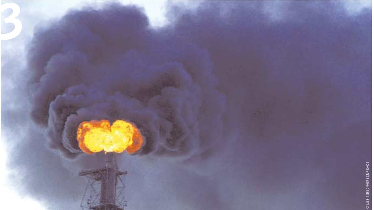
image FLARE STACK AT AN OIL REFINERY IN IMMINGHAM, UK.
